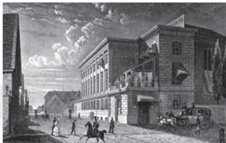
Today's Historic Chemical Landmark site in 1867.
